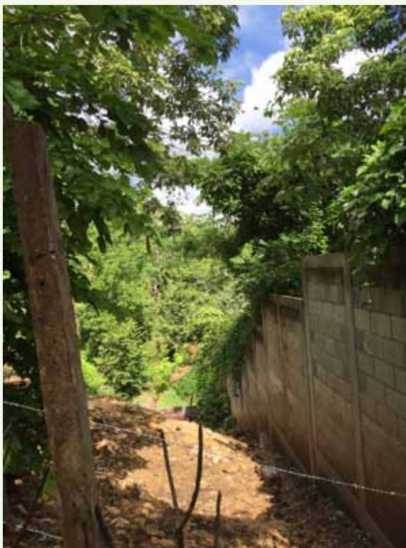
Fencing crossing El Ceibo town, path used by migrants
